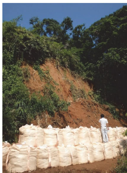
Large sandbags in the front part (from the southeast) (Photo provided by Uto City)
