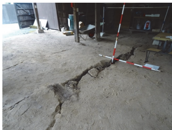
The ground crack in the barn
