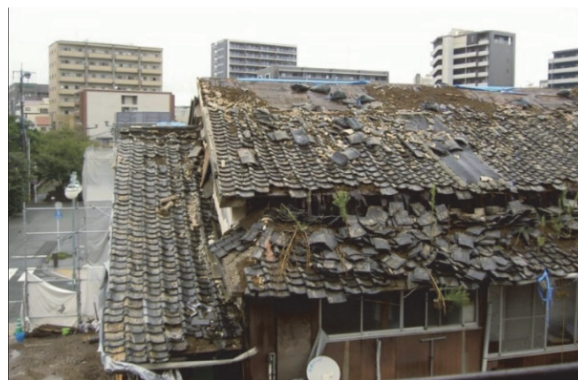
Damage to the main roof
