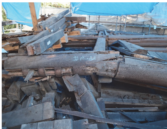
Damage condition: fallen posts
