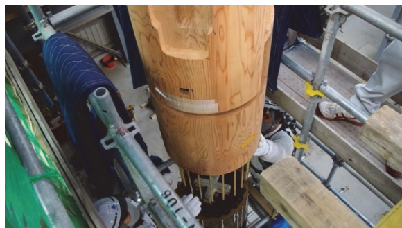
Joints at the top of the posts using aramid rods
