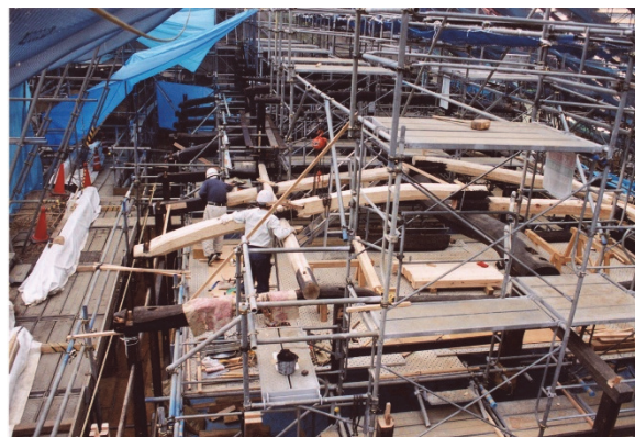
Figure 5.2.2 An example of repair of damaged parts: replacement and maintenance of damaged beams in minka (folk houses)
