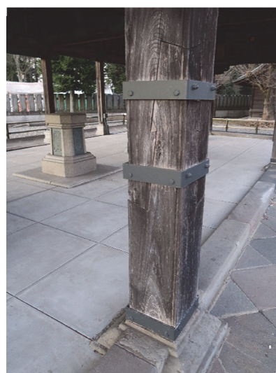
Figure 5.2.13 Metal plate bands reinforcement placed around a post
