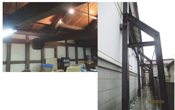
Steel buttress and truss reinforcement to increase horizontal rigidity in the former sake brewing warehouse and sake starter house
