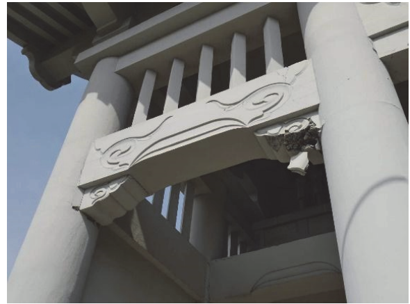
Damage to the column head, intermediate beam, and elbow section (east side: south side)
