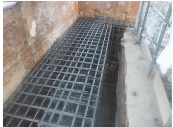
Reinforcement of horizontal structure in catwalk area
