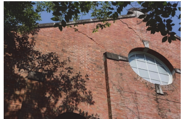
The Experimental Factory for Mechanical Engineering, cracks entering at an angle from the round window in the gable wall
