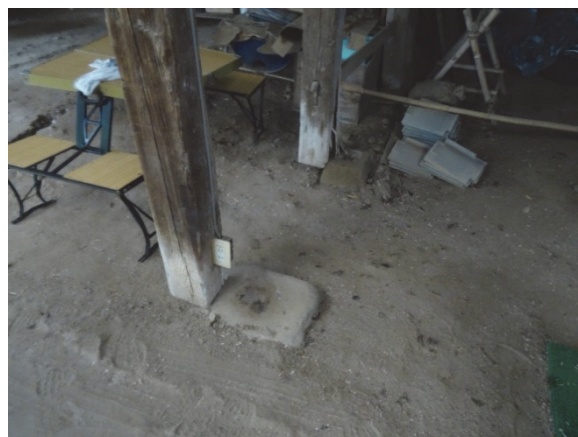
The displacement of the frame post and the foundation stone
