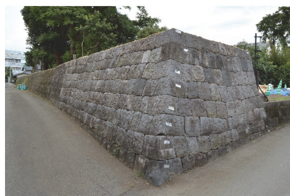
Stone wall reinstallation completed
