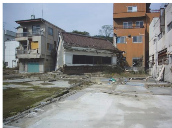
The tsunami swept the first floor away and pushed the second floor about 30 m north
