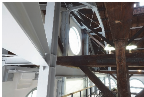
The experimental factory for mechanical engineering, steel reinforcement after the recovery
