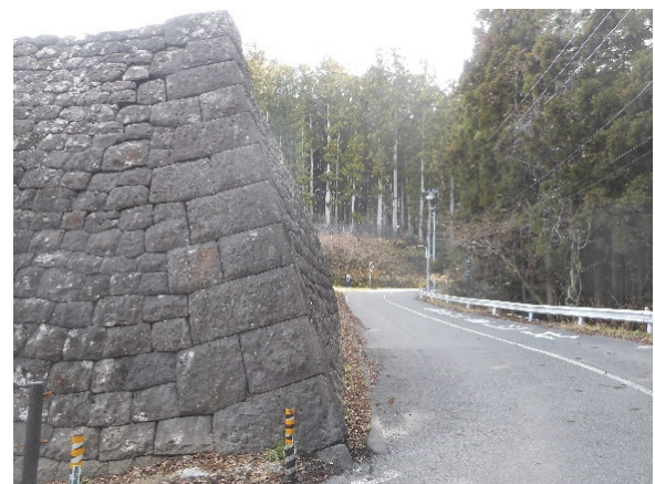
Deformation of the C-side stone wall northwest of the central compound caused by the Earthquake off the coast of Fukushima Prefecture in 2022
