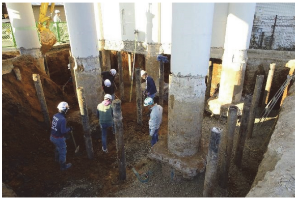
Underground conditions (column bases, footings, cast-in-place piles, additional steel pipe piles)
