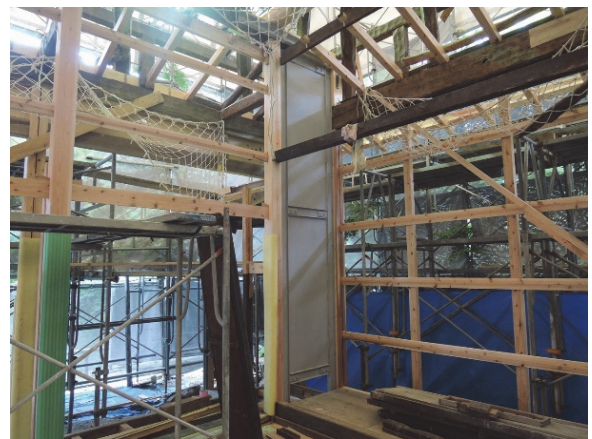
Structural reinforcement example, steel framing
