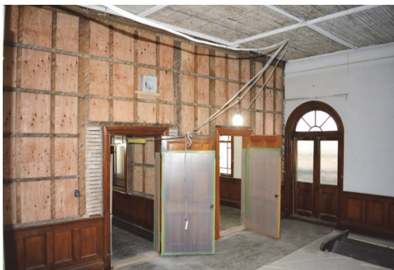
Figure 5.2.4 Structural plywood wall used for reinforcement
