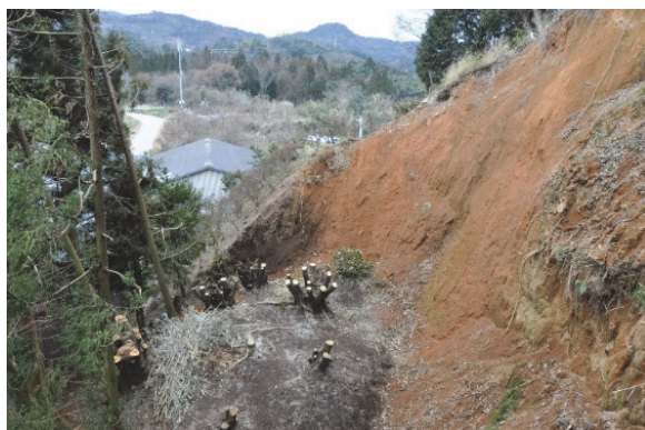
Collapsed soil in the back circle section (from the east) (Photo provided by Uto City)
