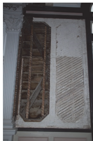
Diagonal braces inside the wall
