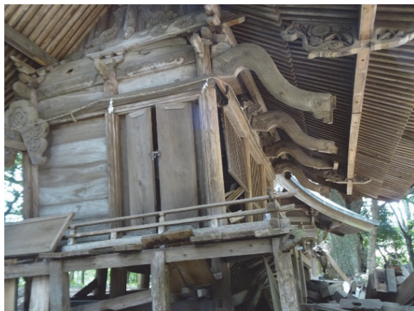
Damage right after the earthquake: Hachio-sha Shrine main frame
