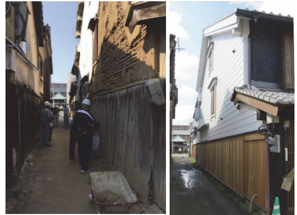
Damage to the alley side wall (left) and after restoration was completed (right)
