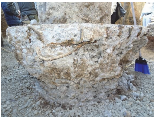
Reinforcing steel bars in the footings and piles driven in place directly under the footings
