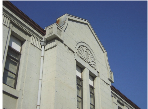
Damage of the pediment
