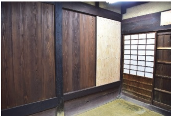
Figure 5.2.3 Seismic fixtures and fittings
