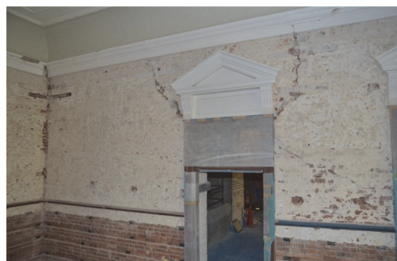
Wall cracks in the Office Building
