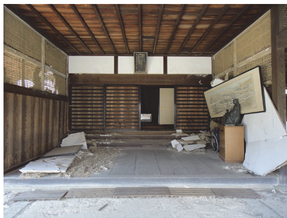
Damage of plaster walls in the carriage porch
