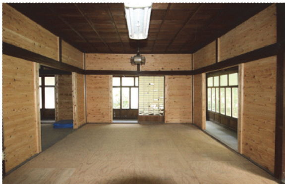
Additional cedar plank earthquake-reinforced walls in the study room
