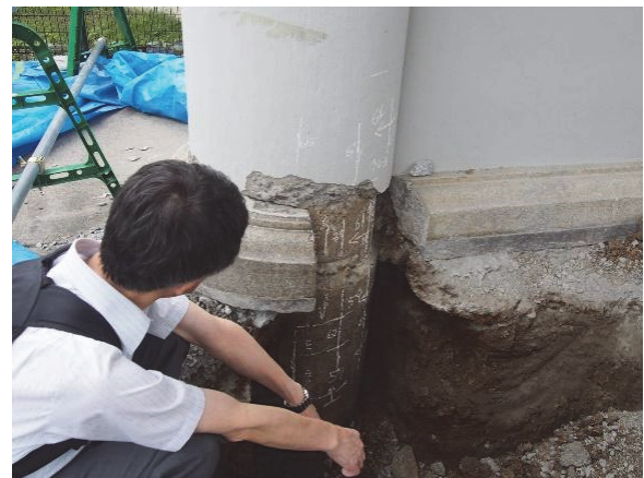
Underground conditions around the column bases (columns in the northwest corner) (Photo courtesy of Mariko Nishijima)
