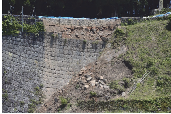
Collapsed stone wall due to heavy rain
