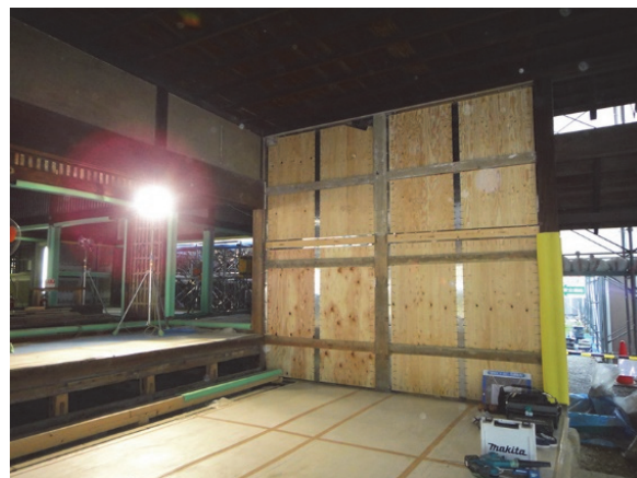
Retrofit with structural plywood plates in the carriage porch
