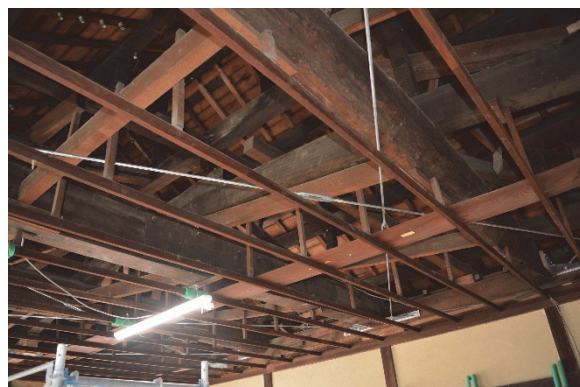
Figure 5.2.10 Horizontal structure reinforcement with steel bar braces
