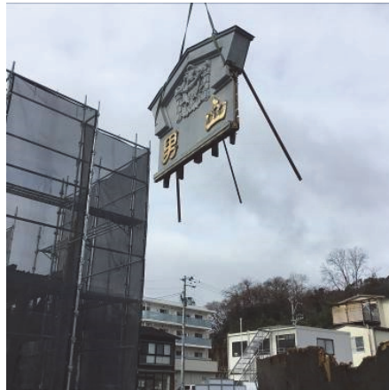
Rescuing the pediment of the third floor to be stored
