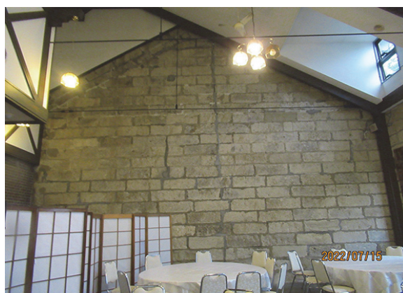
The repeated crack damages by the February 16, 2022, the Earthquake off the coast of Fukushima Prefecture (Former rice storing and milling house)
