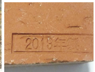
Inscriptions (2013) were made to newly added materials to distinguish them from the original materials
