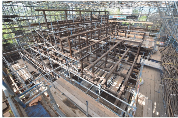
Assembling the main building's earthen floor wing (up to the truss and purlins)
