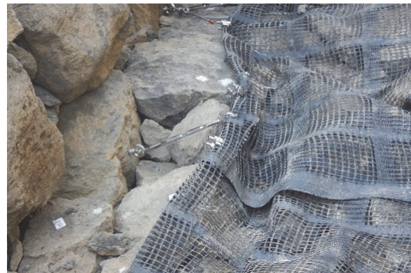
Tightening connections of the geotextile
