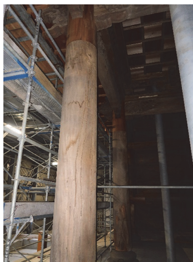
Figure 5.2.17 An example of earthquake resistant measure using inorganic material (Aramid rods). Only the upper part is a new material that is jointed to the original post. (Aso Shrine)
