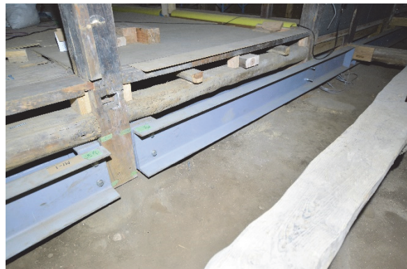
Channeled steel hardware installed for reinforcing column legs at the boundary between the earthen floor and tatami floor wings
