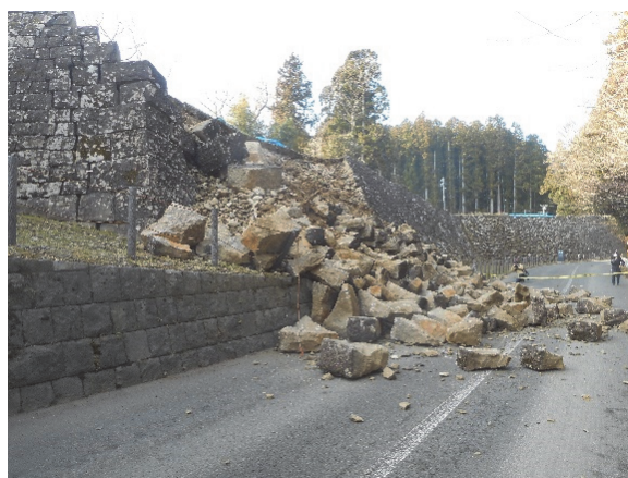
Northwest stone wall E-side of Central Compound (Main Compound) that collapsed again after the Earthquake off the coast of Fukushima Prefecture in 2022
