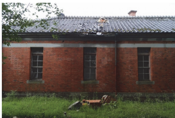
Chemical Laboratory, the broken and fallen chimney
