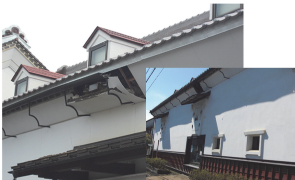
Former sales warehouse (inclined building and damaged eaves)
