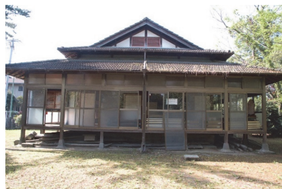
Overall view after the earthquake (the building was not so rigid that the shaking did not dislodge the foundation strut stones)
