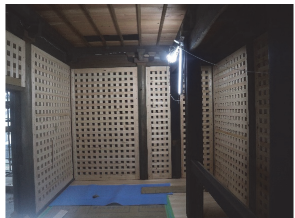
Reinforcement latticed walls over the floor
