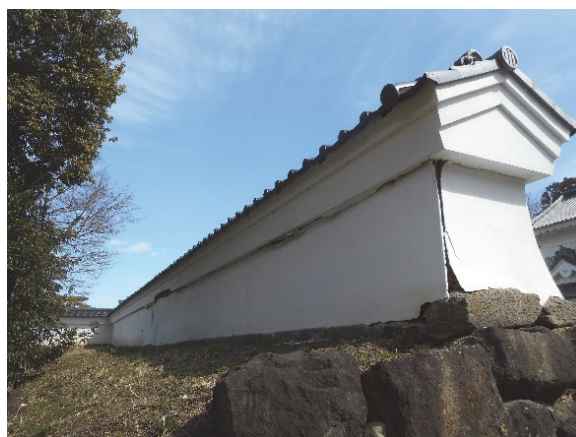
Earthen wall on the north side of the Otemon gate deformed by the Earthquake off the coast of Fukushima Prefecture in 2022
