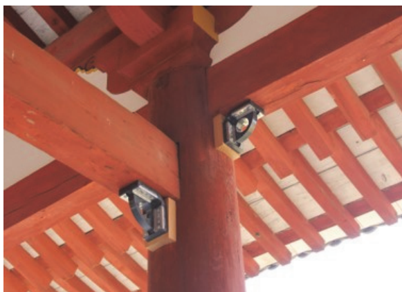
Figure 5.2.9 Seismic reinforcement ring made of resin
