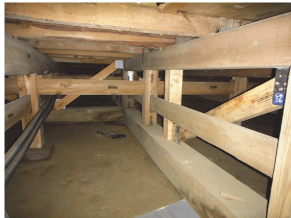
Diagonal bracing reinforcement under the floor
