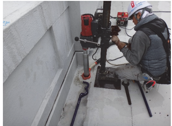
Insertion of deformed steel bars into brick wall
