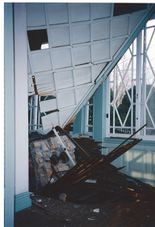
Photo 2.12 An example of a chimney that fell indoors (Former Hunter Residence) (Photo provided by Agency for Cultural Affairs)
