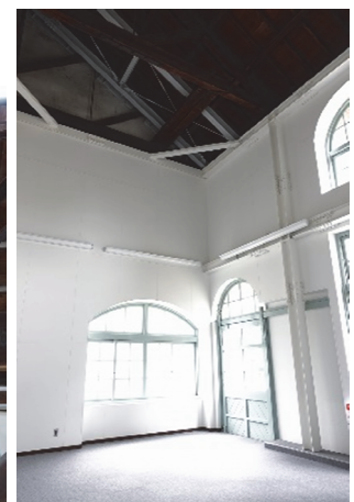
The experimental factory for mechanical engineering, steel reinforcement after the recovery
