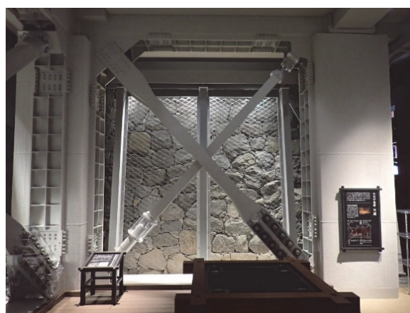
Seismic reinforcement (cross damper) in the Tenshukaku castle towers
