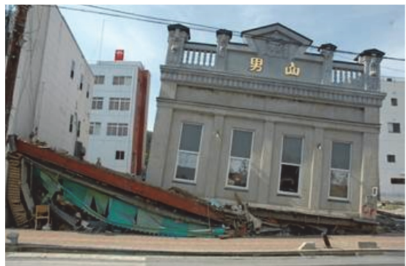
The tsunami swept the first and second floors away, leaving the third floor
