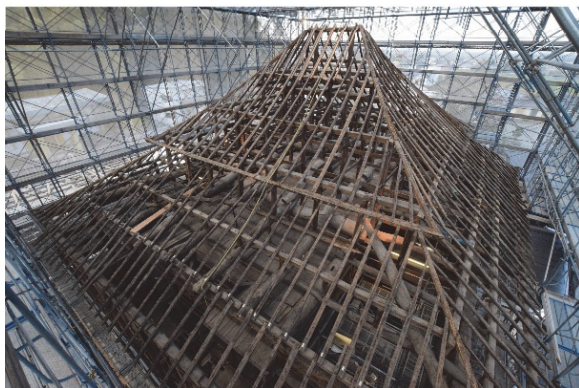
Roof dismantlement in progress, Kaijo-ji the main hall, view from the northeast
