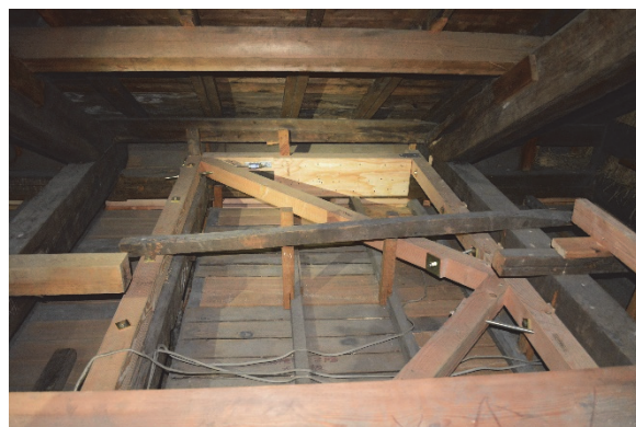
Figure 5.2.11 Reinforcement to horizontal structure with wooden braces
