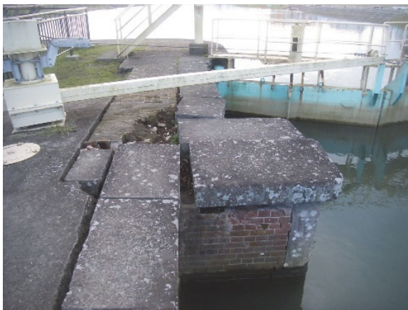
Damage conditions of the gate posts at the lock tail (left bank) after the switch gate was replaced
