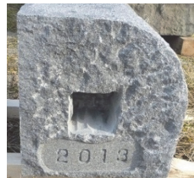
Inscriptions (2013) were made to newly added materials to distinguish them from the original materials
