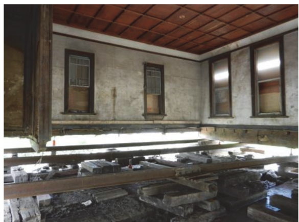
Preparing the rails to roll and move the remaining building part
