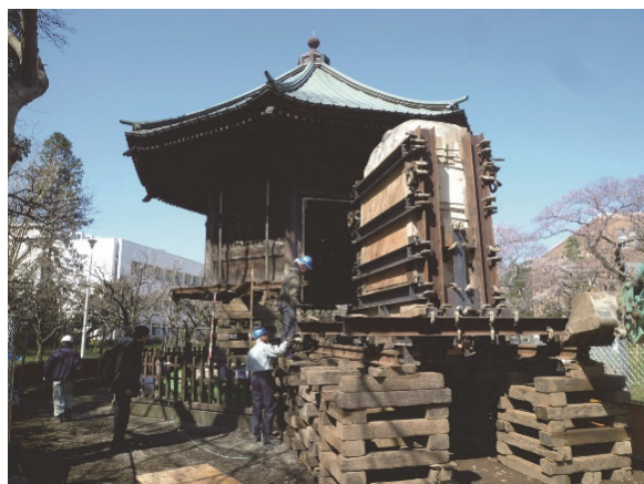
The body of the monument was lifted and moved on rails
