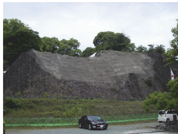
Stone wall of the Higashi-Juhachiken-yagura turret (after dismantling)
