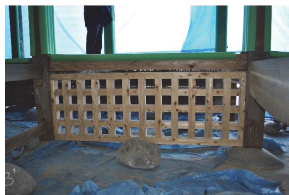
Figure 5.2.14 An example of reinforcement under the floor
