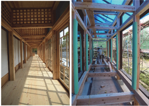
Reinforcement by lattice wall (Add lattice grid at the top opening section. The footing is rigid and takes up a lot of strength.)
