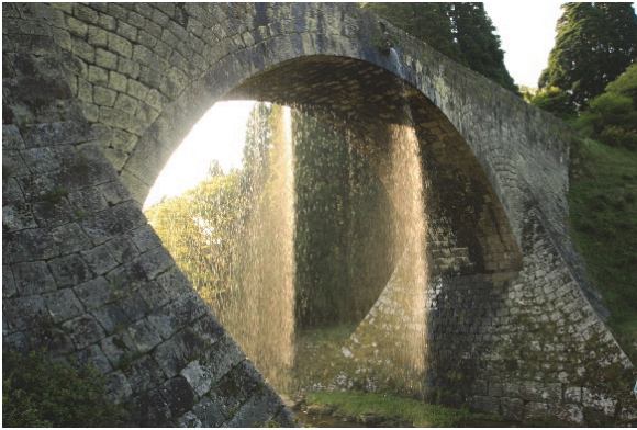
After the earthquake, leakage from the arch bridge
