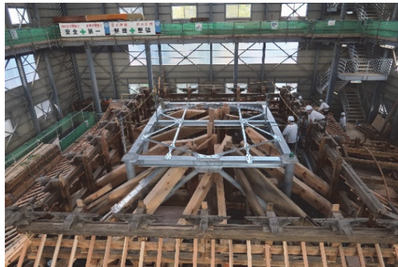
Steel Seismic Reinforcement Frames and Dampers, Tower Gate interior
