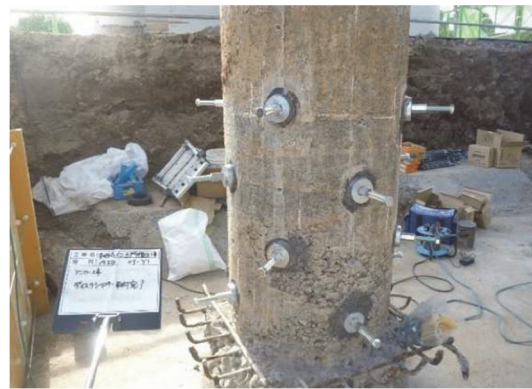
Disc shear key to join the columns to additional footings (Photo courtesy of Den Arch.& Eng. Office)
