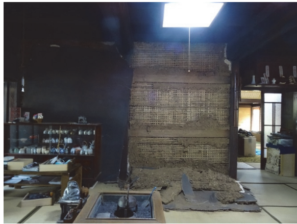
Collapsed living room interior wall of the main building
