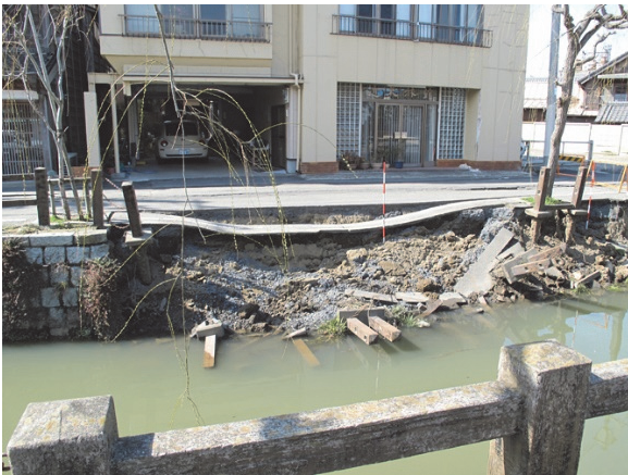
Damage to the revetment in the preservation district (Photo provided by Katori City)
