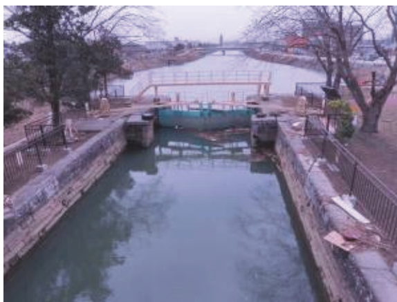
Damage conditions of the lock chamber and lock tail after the tsunami
