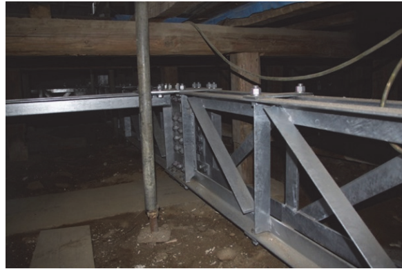
Subfloor steel beam
