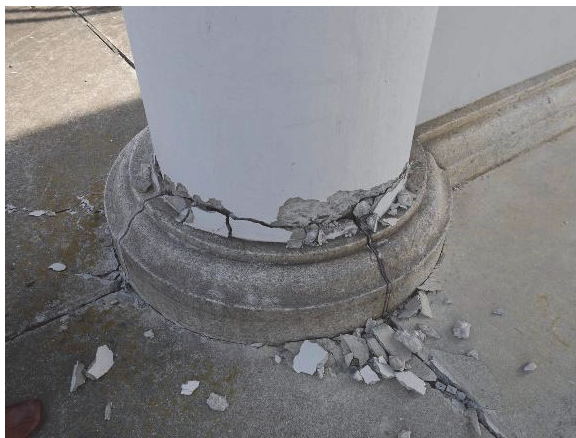
Damage near column bases (columns in the northwest corner)
