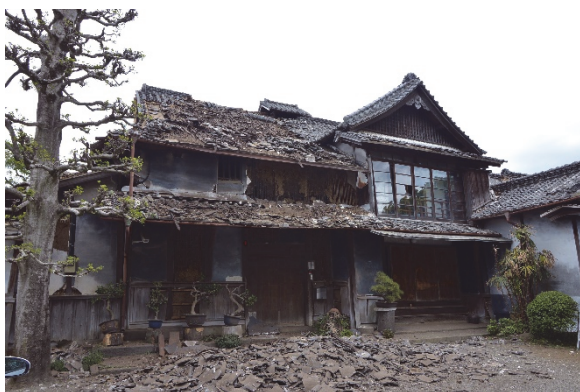
Damage to the main building: South front (West side tiles have fallen. The frame is largely tilted.)
