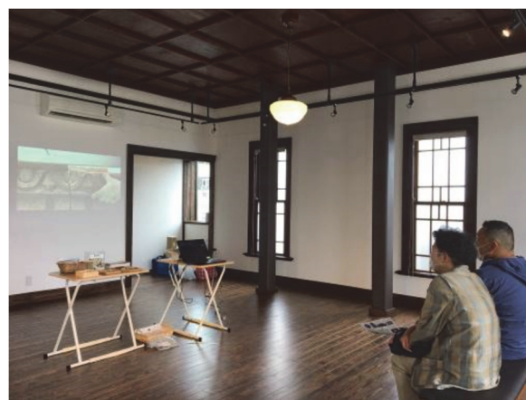
New reinforcement steel columns were installed to retain the open space of 8 m
