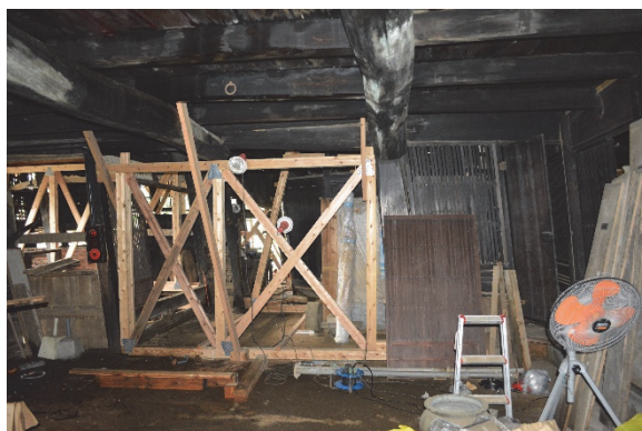
Figure 5.2.15 An example of emergency measures: installation of braces
