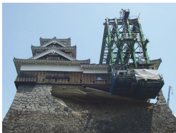
Preventing the Iidamaru-Gokai-yagura turret from collapsing
