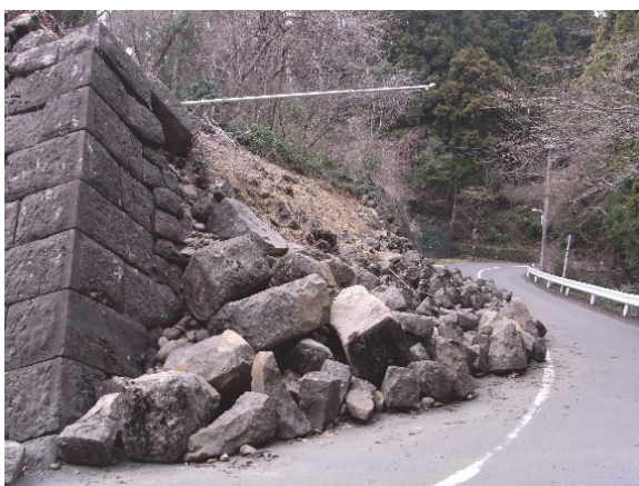
The c-side of the northwest stone wall of the central compound collapsed due to the Great East Japan Earthquake in 2011
