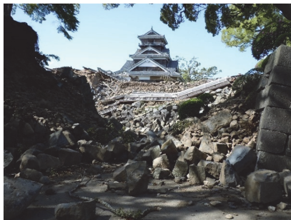
Damage to stone walls
