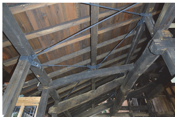
Horizontal braces installed on the north roof of the earthen floor wing
