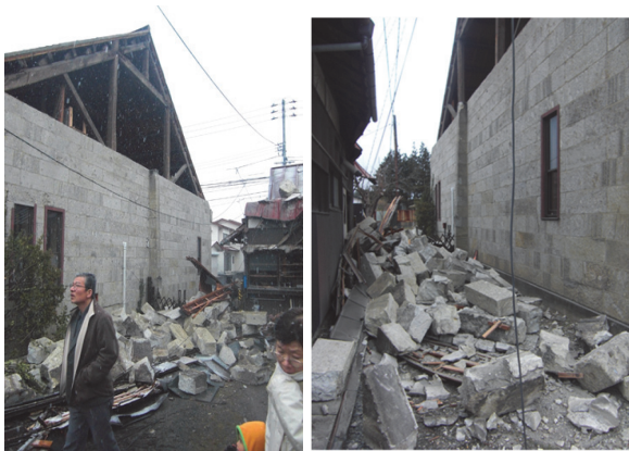
Former rice storing and milling house (collapsing stone walls)
