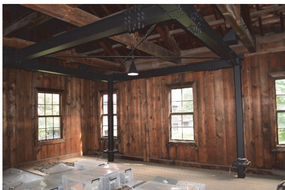
Figure 5.2.8 Steel frame reinforcement
