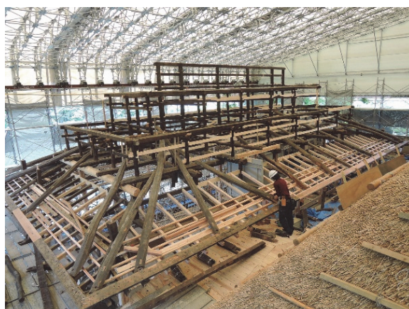
Erecting of floor frames, posts, and truss
