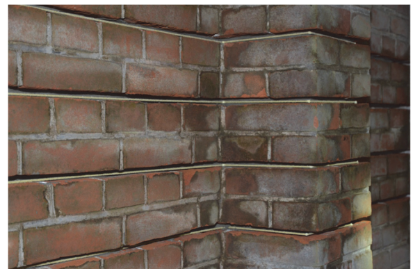
Reinforcement of the joints, Office Building
