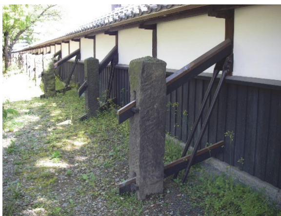
Reinforcement to the stone pillar supports of the Nagabei wall
