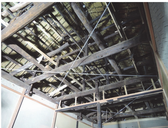
Roof truss with iron rod bracings
