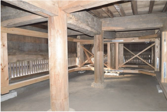
Wooden staff reinforcement under the Shrine floor
