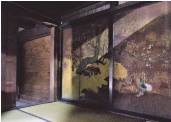
Installed cedar plank earthquake-reinforced walls (left side of the board door)
