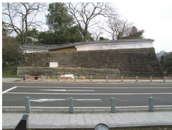
Earthen wall on the north side of the Otemon gate collapsed by the Great East Japan Earthquake
