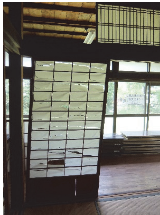
Estimated to have shaken up to 1/12 radian based on residual deformation of the shoji
