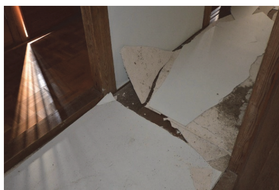
Interior of the building after the earthquake (collapsed wall top coat)
