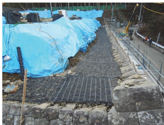
Geotextile reinforcement work at the C-side of the northwest stone wall of the central compound
