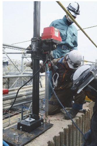
Drilling holes in the masonry wall
