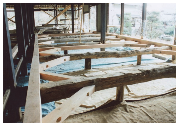
Figure 5.2.12 Under the floor reinforcement
