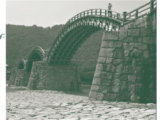
Kintaiyko Bridge (Iwakuni, Yamaguchi pref.)
