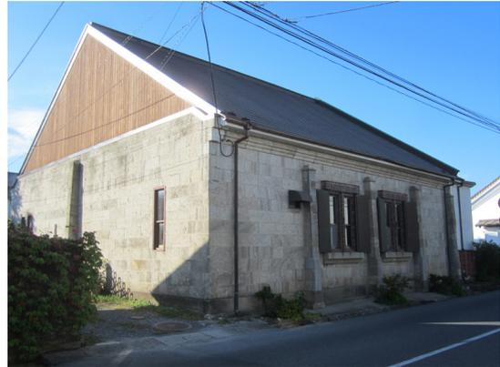
Figure 2.23 Wooden boards were placed as an emergency measure for the collapsed wall
