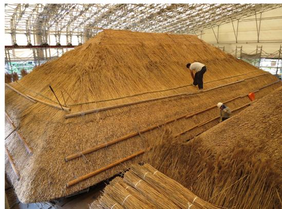
Figure 2.9 Roof thatching
