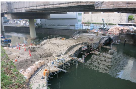
Figure 2.29 Dismantling of the bridge
