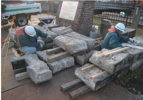
Figure 2.31 Dismantling and custody of the stone blocks
