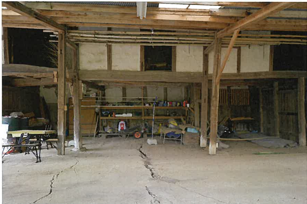
The crack in the barn of a Yano Residence, Nishihara Village, Kumamoto Prefecture
