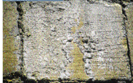
Porous limestone, salt crust (halite).
