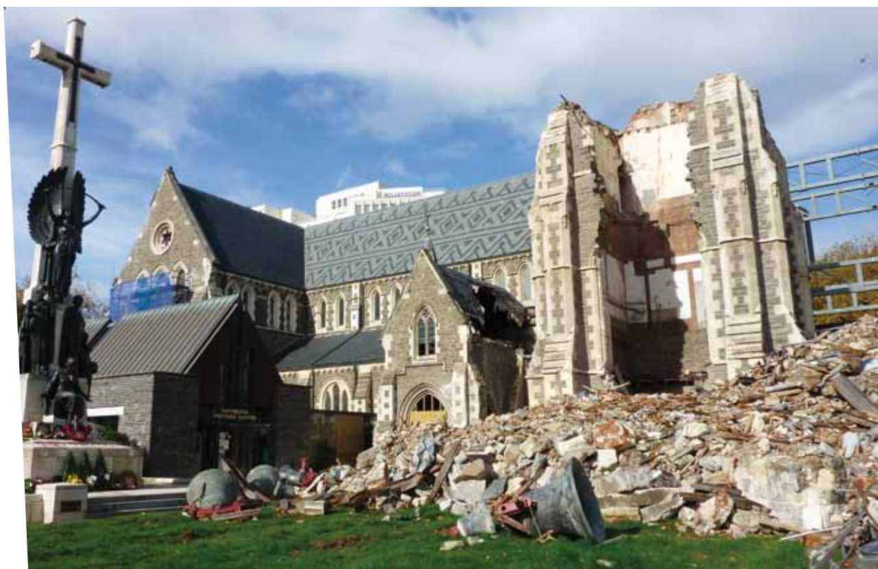
Bells and debris from the spire of Christ Church Cathedral, consecrated in 1881, lie in Cathedral Square. Steel shores on the right support the west wall and the rose window. The February quake cracked pillars, twisted walls, shattered stained glass and collapsed buttresses.
