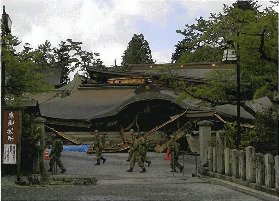
The collapsed Romon gate of Aso Shrine, Aso City, Kumamoto Prefecture
