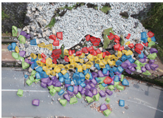
Figure 3.7.1.10 The collapsed Miyauchi dry stone wall
