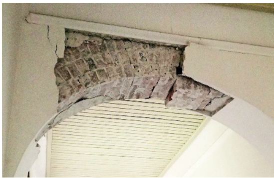
Photo 3.2.2.3 Cracks and fall down of the surface plaster on the corridor arch. (The Fifth High School Main Building)
