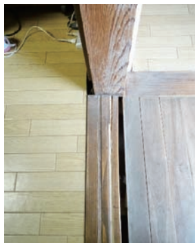
Photo 3.1.2.7 The thresholds have become misaligned at the main building of the Yano family home ( Hontaku )
