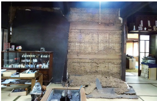
Photo 3.1.2.5 The wall of the formal room collapsed at the main building of the Yano family home ( Hontaku )
