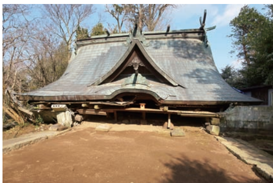
Photo 3.1.5.1 The remaining roof of worship hall of Kiyama Shrine after the earthquake.
