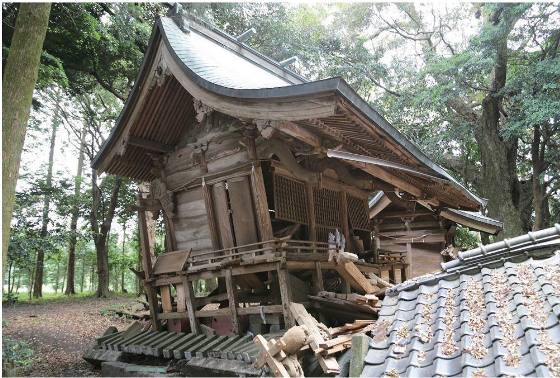
A huge sloping the main hall and collapsed the worship hall, Hachiosha Shrine
