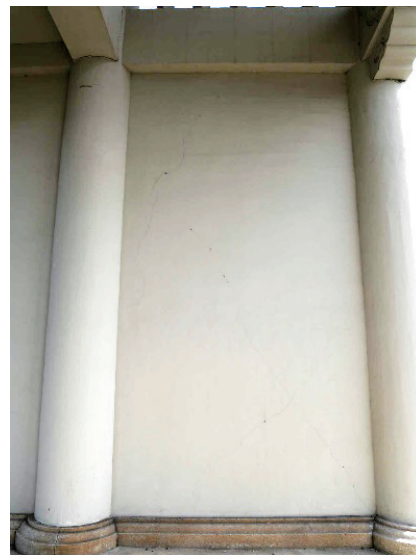
Photo 3.3.1.6 Honmyo-ji Nio-mon: shear cracks in the walls.
