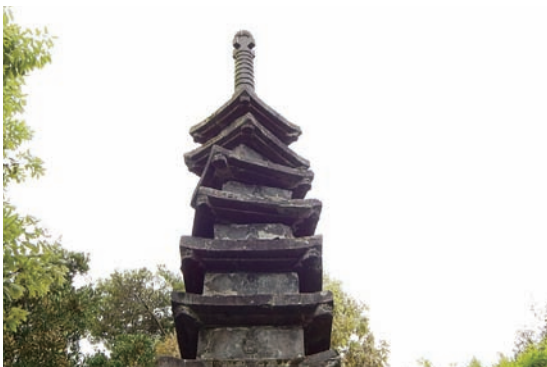
Photo 3.6.2.2 The upper part of the twisted thirteen-storied pagoda
