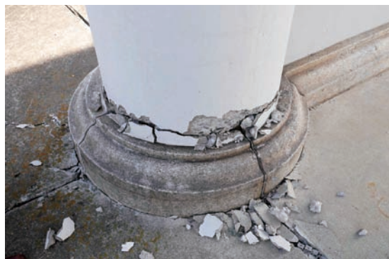
Photo 3.3.1.4 Honmyo-ji Nio-mon: damage to a column base.
