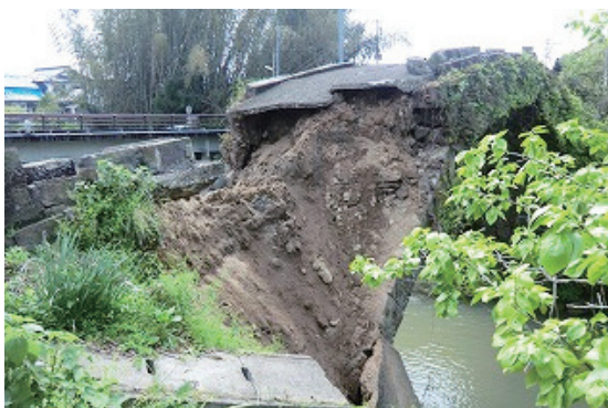
Photo 3.6.1.5 The stone wall collapsed at the Yasumi-shimoduru Bridge (Photo by Uki city)
