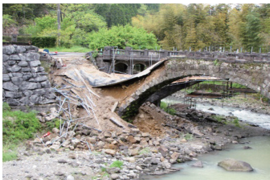
Photo 3.6.1.2 The collapsed stone wall at Futamata Fuku-ura-watashi
