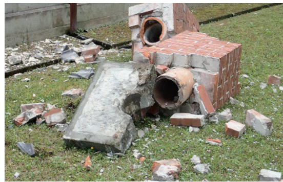
Photo 3.2.2.4 Fragments of a chimney on the ground. (The Fifth High School Chemical Lab.)
