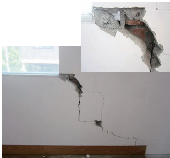
Photo 3.2.1.3 Cracks appeared around the openings.
