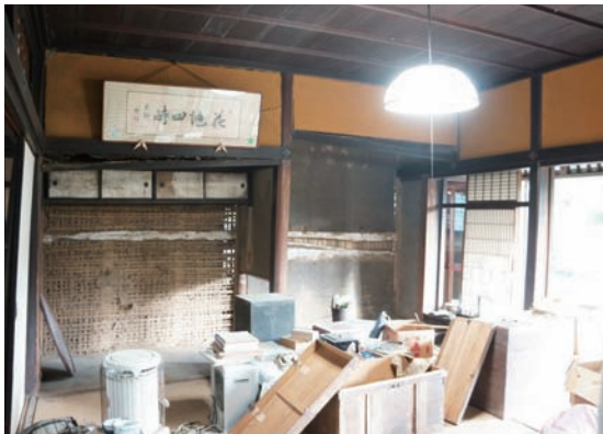
Photo 3.1.10.5 The sitting room: Collapsed interior earth wall.
