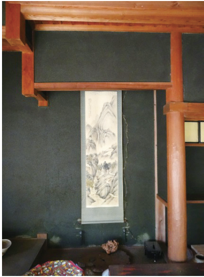
Photo 3.1.2.13 A fissure in the wall of the alcove of the Yano family home ( Shintaku )
