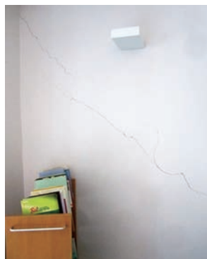
Photo 3.2.1.4 Shear cracks appeared in the walls.
