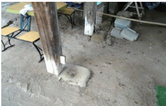
Photo 3.1.2.3 The shed pillars have come off their foundation stones at the Yano family home ( Hontaku )
